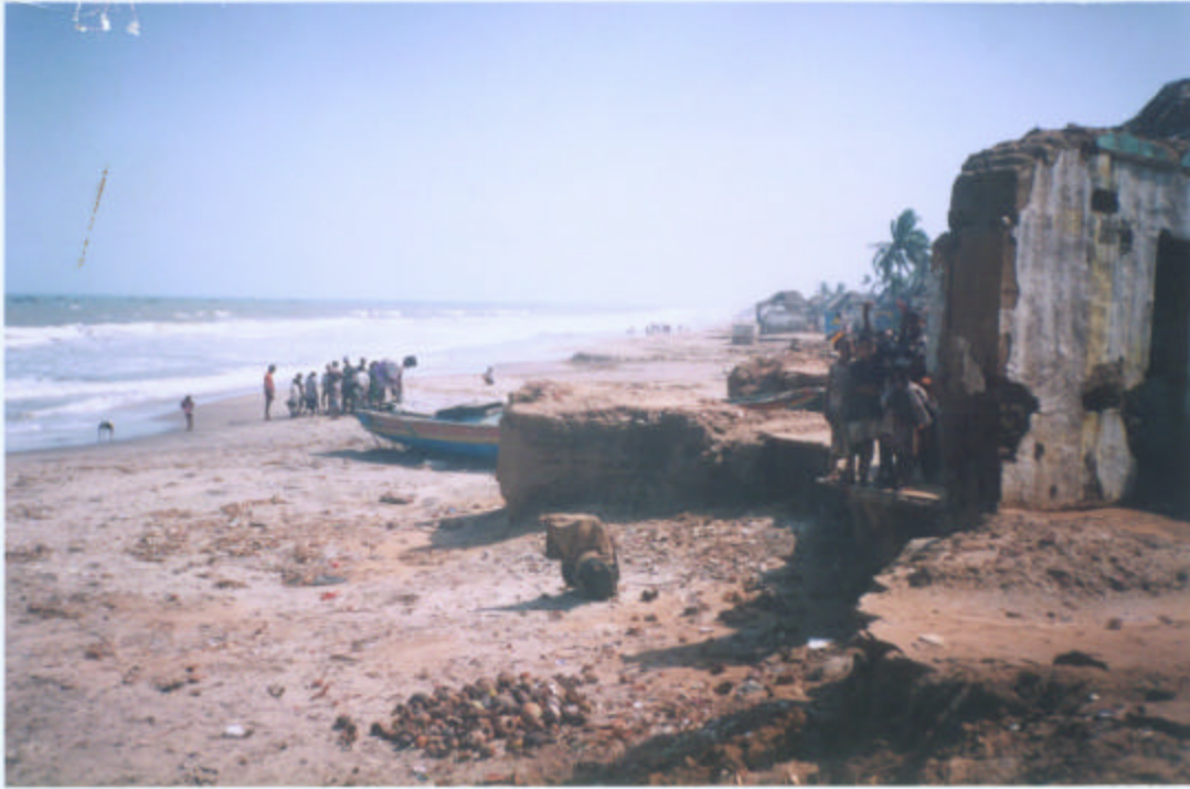
PHOTO SHOWS EXTENT OF SEVERE EROSION AT UPPADA
