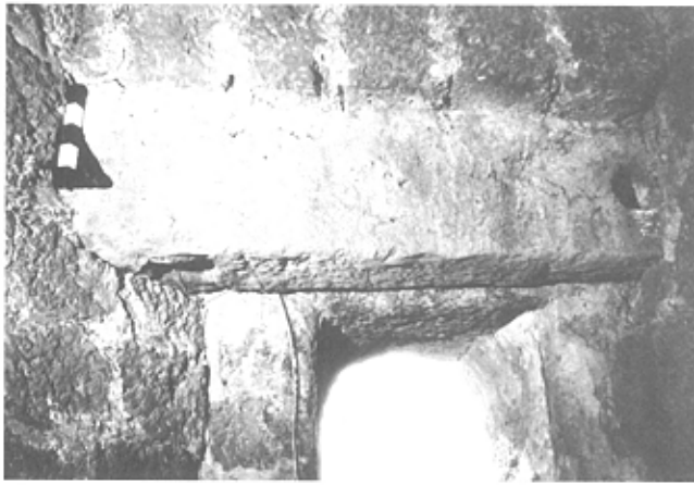
Figure 16. Grapnel stone anchors noticed as lintels on the arches of the parapet wall of the second fortification of Vijaydurg Fort. (Photo: S.N. Bandodkar) Scale in 5 cm units.
