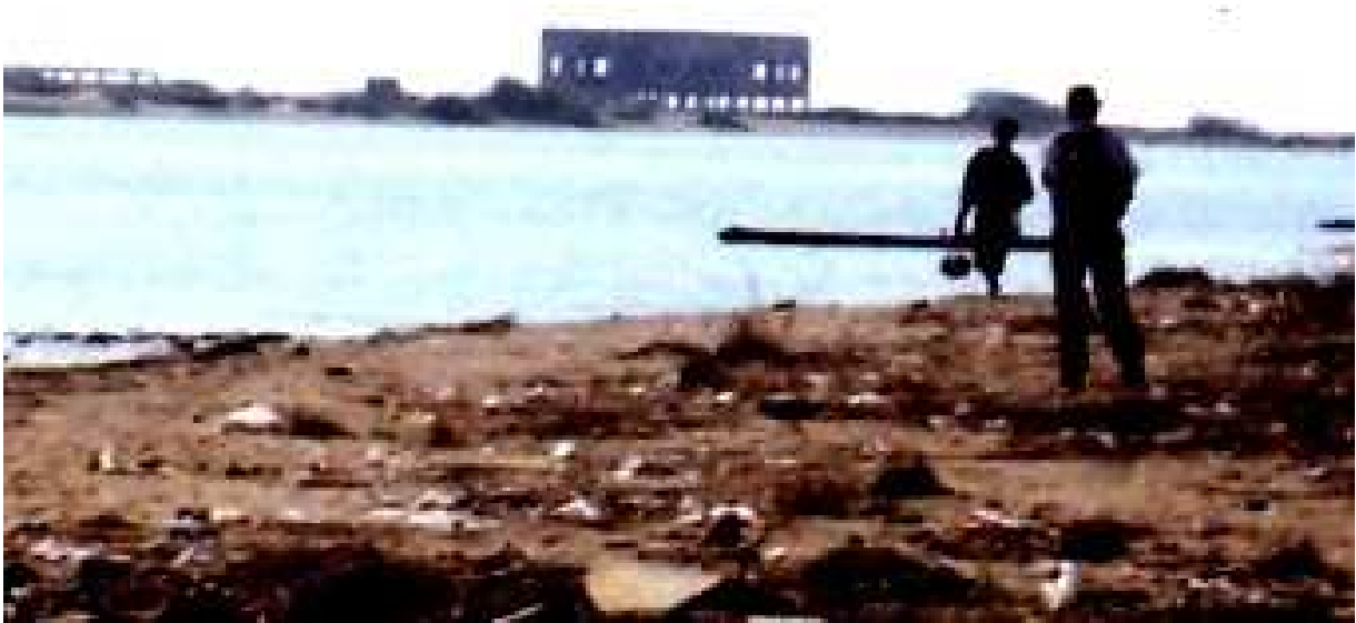
Plate 17. A concrete structure on stilts built right on the beach but remained unaffected by tsunami (Tirumullaivasal).
