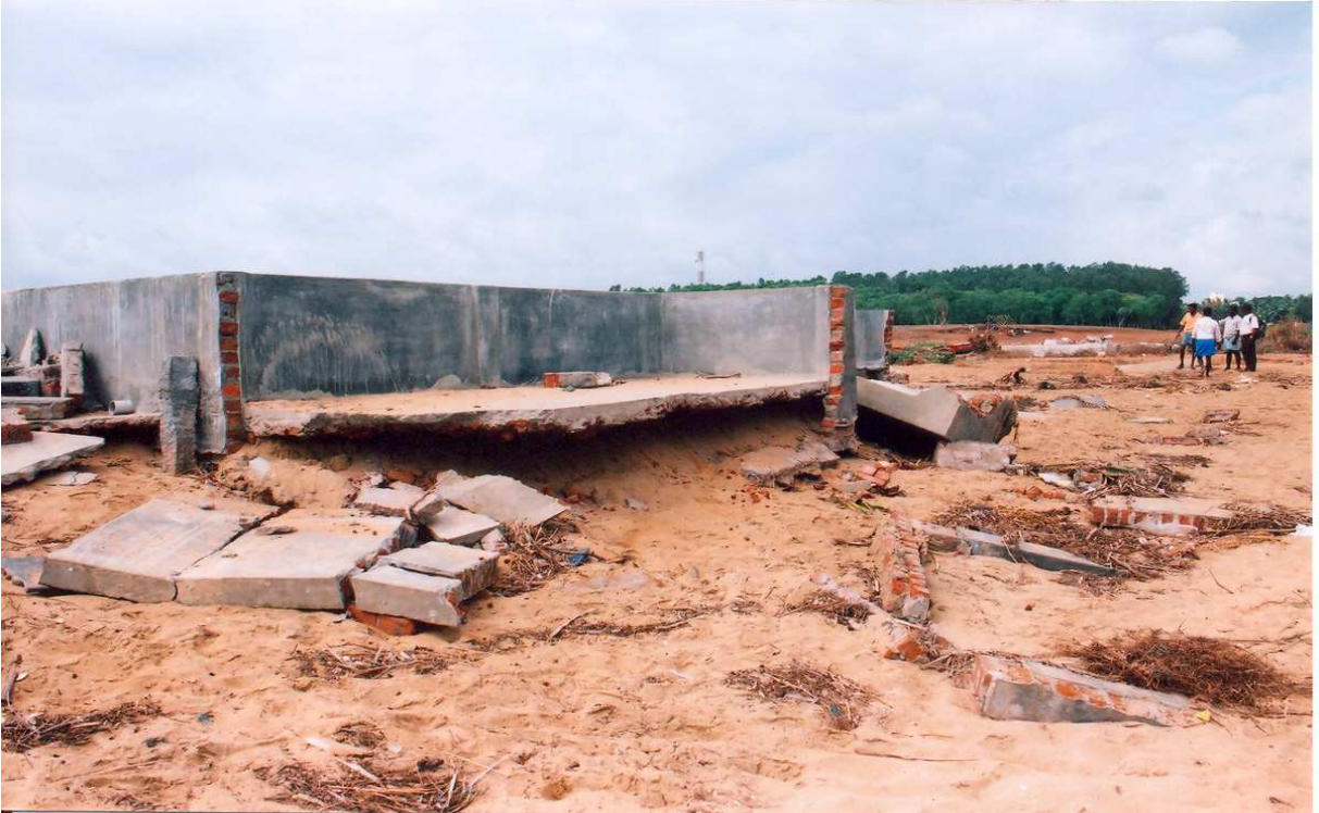
Plate 23. Tsunami damaged structures founded on loose sandy soil (Periyakalpet).
