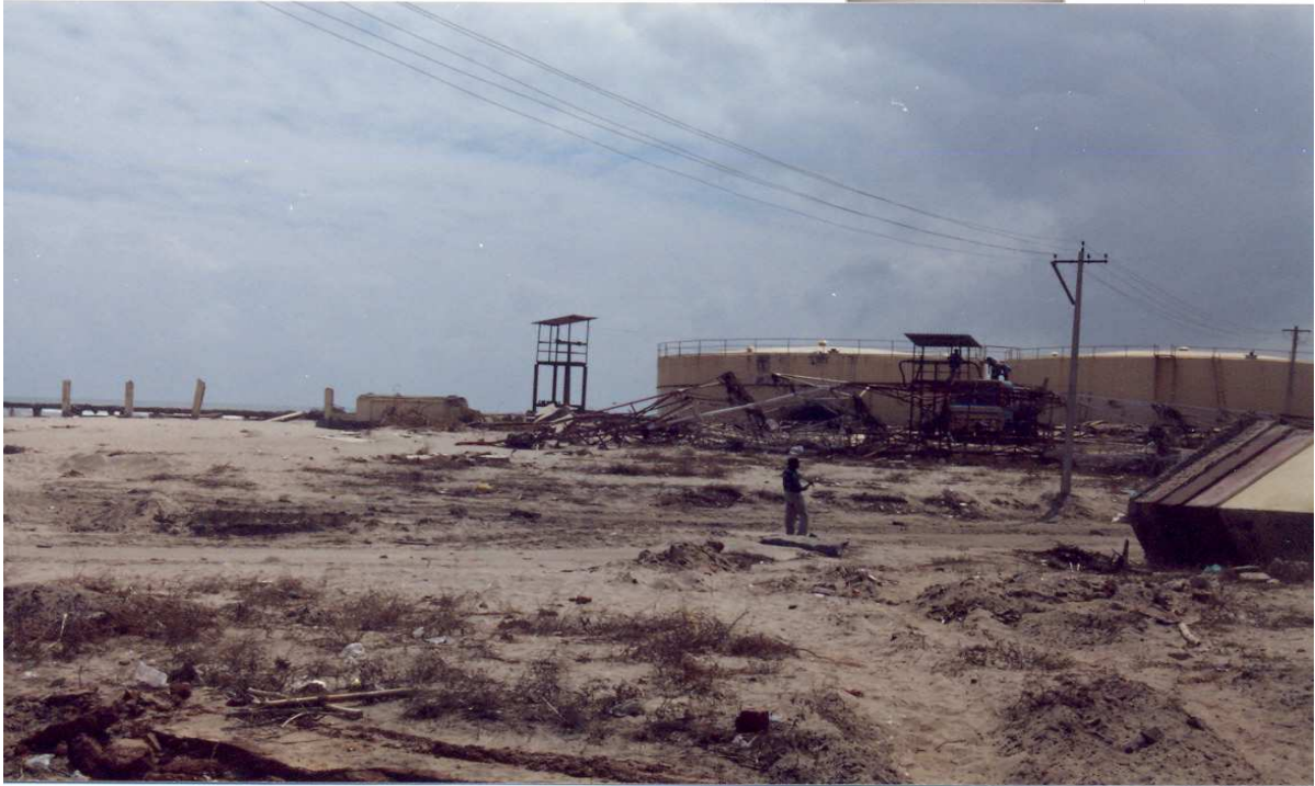
Plate 15. Minimally affected large cylindrical oil storage tanks in the background and the damaged small generator room in the right side (Nagapattinam harbour).
