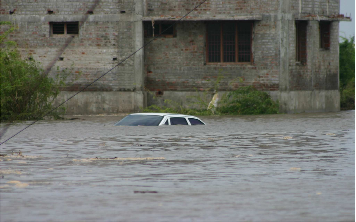
Plate 21. Example of unaffected house built on elevated plinth in the low lying areas (Karaikal).
