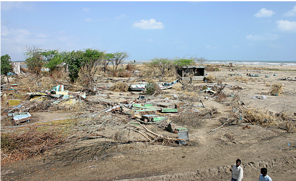
Plate 8. Structures with load bearing walls in close proximity to the sea which failed by the tsunami.
