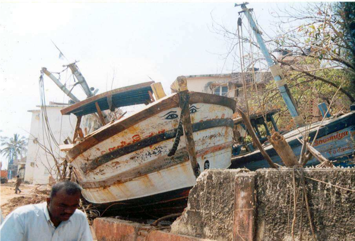
Plate 26. Structures damaged by uplifted fishing trawlers (Nagapattinam).
