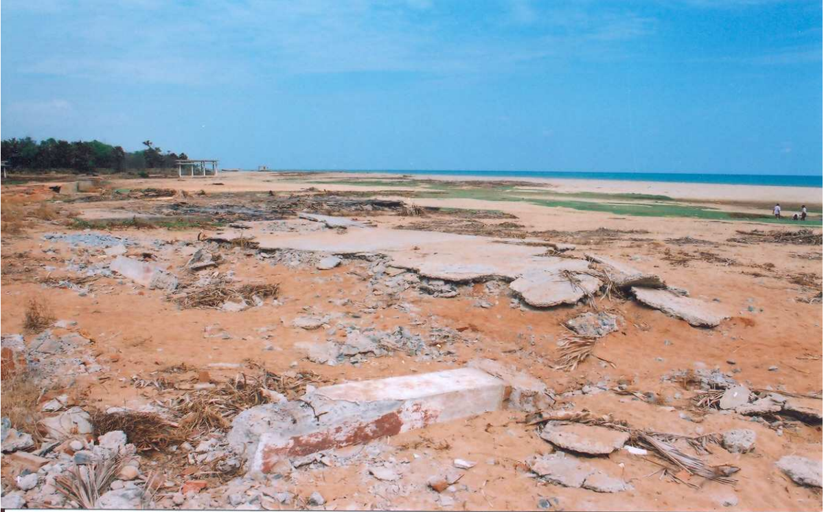
Plate 9. Tsunami damaged inappropriately designed structure built very close to the sea (Periyakalpet).
