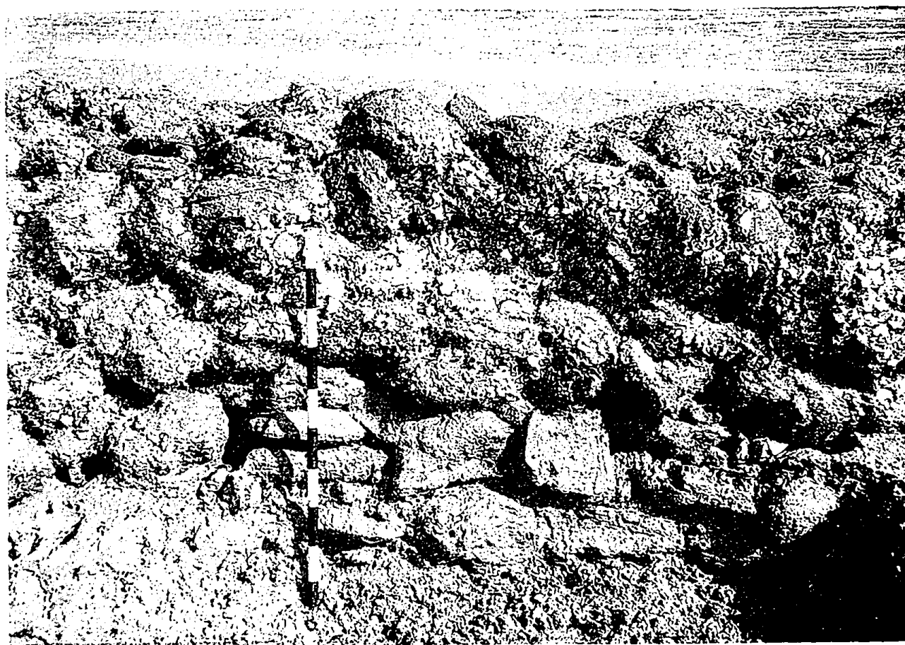
Fig. 32 Section of a trench exposing lower part of rubble wall in BDK VIII
