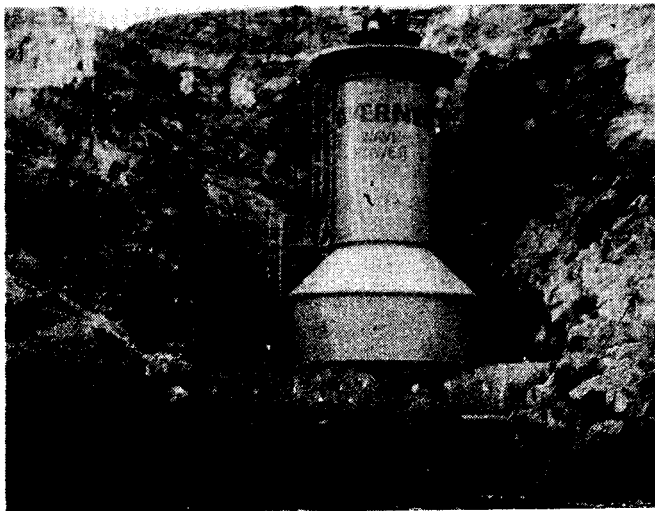
Norwegian wave power plant
