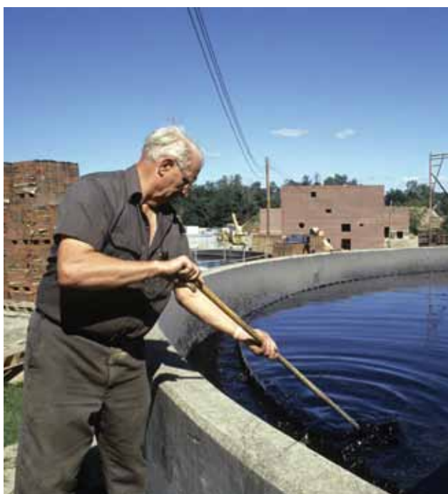
Cleaning the sludge thickener tank at the Water Pollution Control Plant, Danbury, Connecticut, U.S.A.
