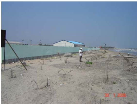
Figure 3: In what appears as a challenge against eventual natural extreme events, the earlier low sea wall (April 2005) that was overtopped by the tsunami, has been extended about 150 meters southward as a taller and broader concrete fortification; beach erosion has already started at the distal end (January 2006). Also note that fear impelled villagers to plant coconut saplings on the beach; these plants perished within a year. The Nagapattinam light house is seen in the background (Photos: A. Mascarenhas and S. Jayakumar, NIO, Goa).
