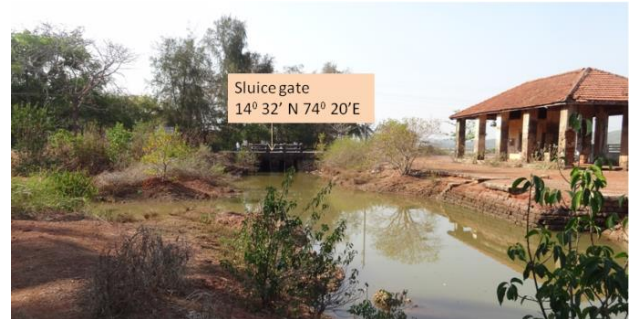
Photograph showing the sluice gate near salt pan at Sanikatta village
