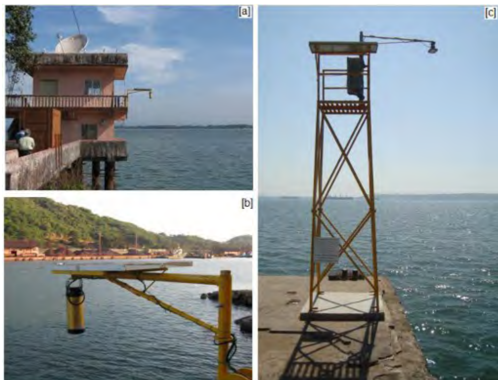
Figure 3. Typical installations of microwave based radar gauges at [a] Karwar, [b] Port Blair and [c] Dona Paula.
